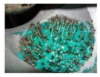
To eliminate or minimize the chance of surface cracks occurring, be careful to finish pouring the resin into the socket until it is just below the tips of the wires, and at or slightly below the top of the socket bowl. Over-topping those tips to provide a smooth even surface may look better initially, but the risk of having the assembly rejected by the customer because of their concern at the site of a crack after proof testing may be a situation you would prefer to avoid.
